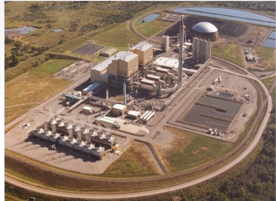
320mw coal fired power plant located near Poteau, Oklahoma
