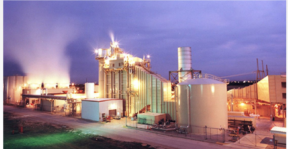
125 MW Combined Cycle unit located in the Oklahoma City metro area
