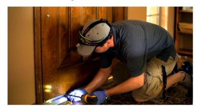
An OG&E crew member provides weather stripping to a customer's doorframe. This process reduces the home's leakage of cool air in the summer, reducing electricity costs and conserving energy for homeowners.
