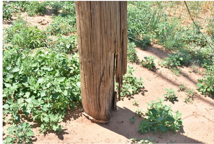
Pole Rot & Groundline Damage
