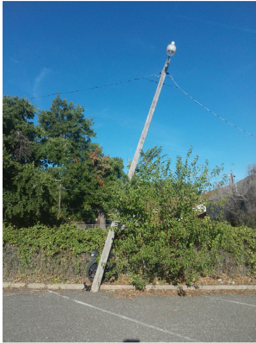
Pole Rot & Groundline Damage
