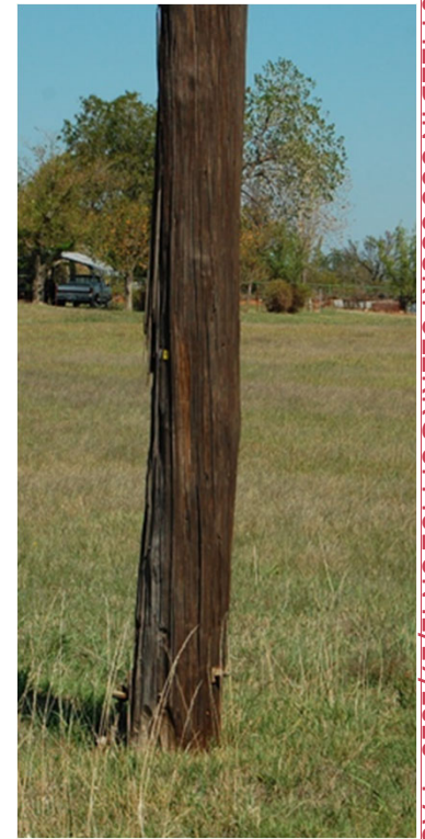
Pole Rot & Groundline Damage
