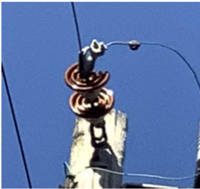
Insulator Damage
