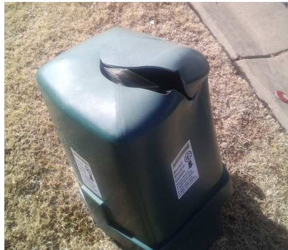
Transformer Damage
