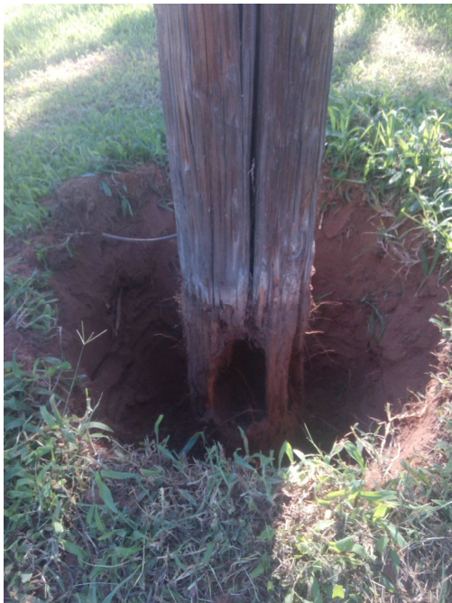
Pole Rot & Groundline Damage
