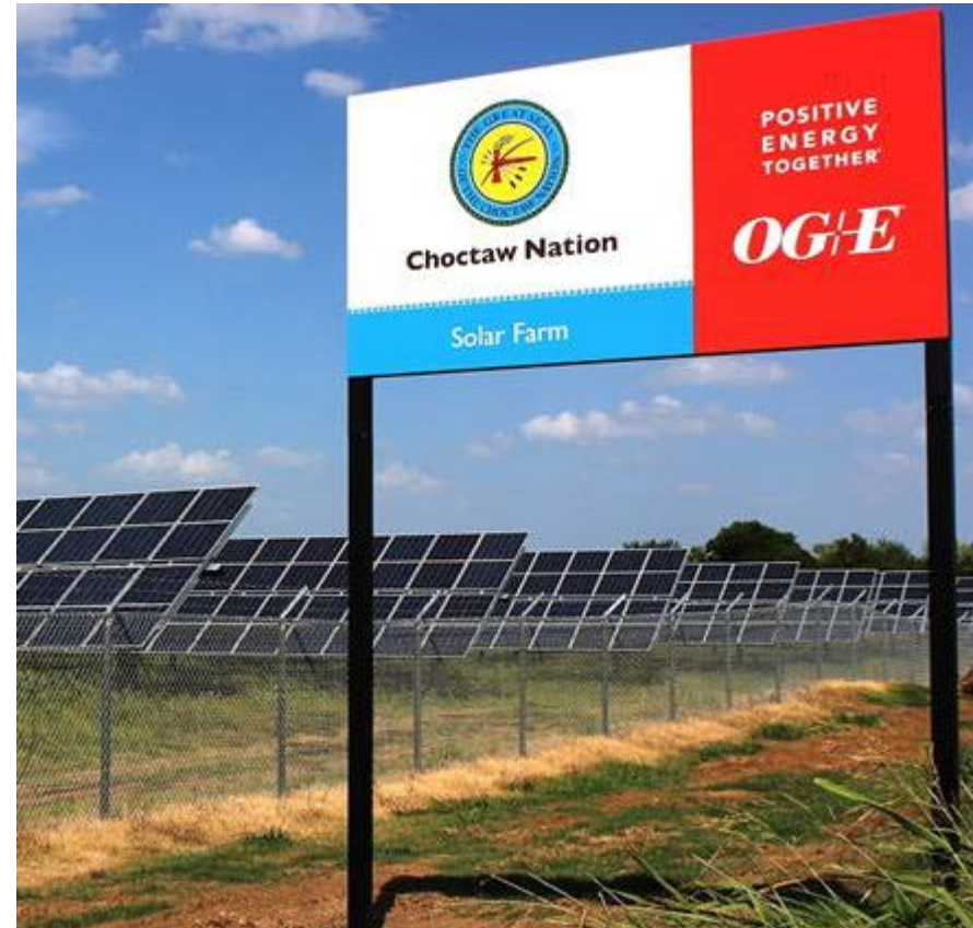
Choctaw Nation/OG&E Solar Energy Center in Durant, Oklahoma
