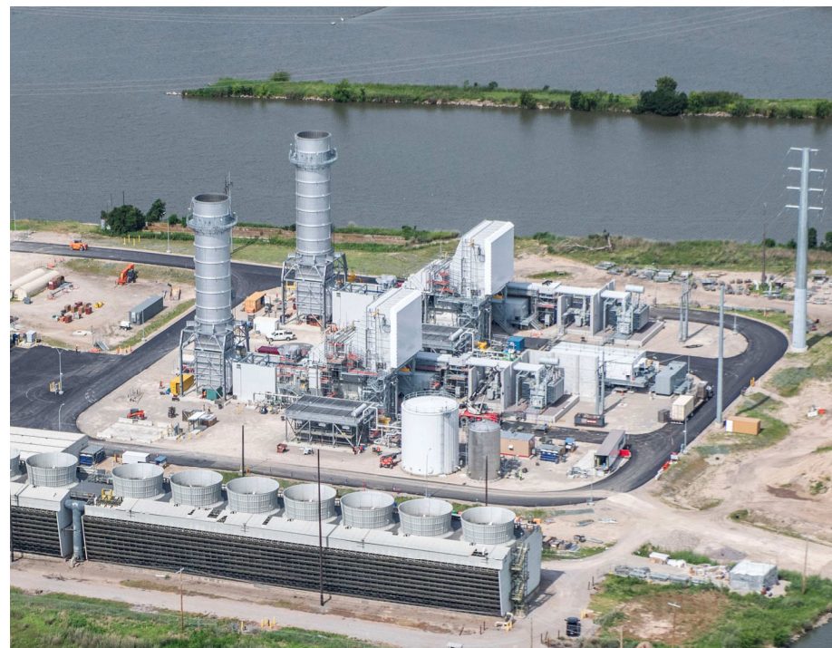
Horseshoe Lake Units 11 and 12 currently under construction with planned in-service date in the second half of 2026.
